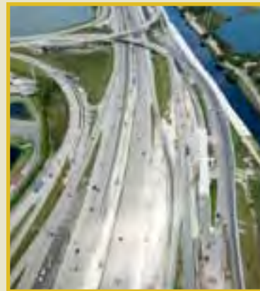
Photo courtesy of the Florida Dept. of Transportation. Florida's I-595 Express is a successful P3 project.
