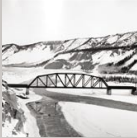
Healy River Bridge
