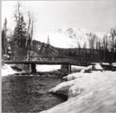
Wagon Bridge at Indian River
