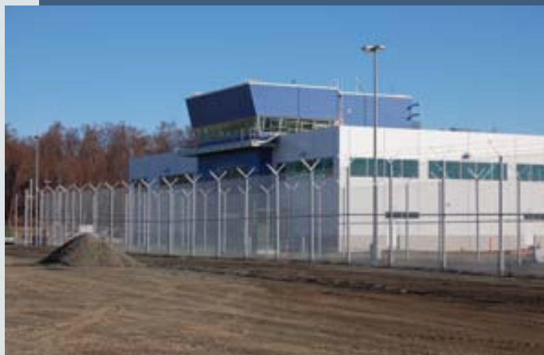
Goose Creek Correctional Center
